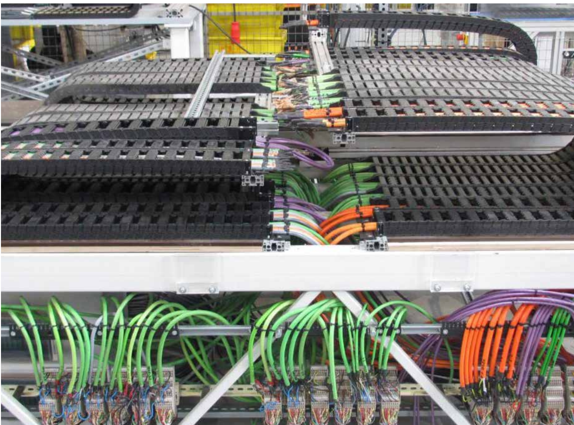
Linear chain tests with continuous monitoring of the electrical cable parameters
